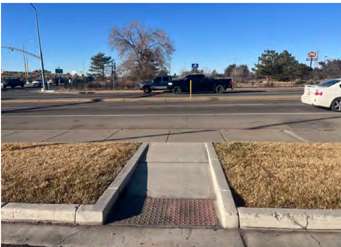
Pedestrian Ramp to the Sidewalk
