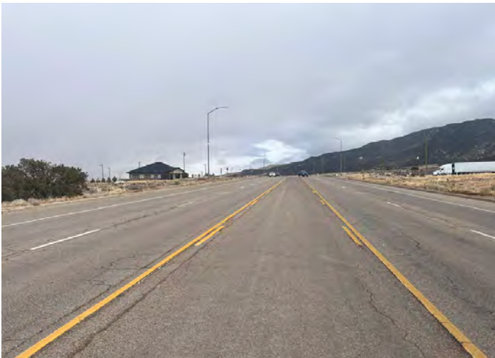
Typical Five-Lane Cross Section, Northbound near Canyon Center Drive
