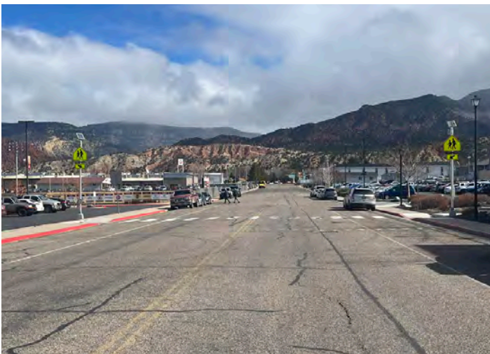
Rectangular Rapid Flashing Beacon Crossing on 800 South
